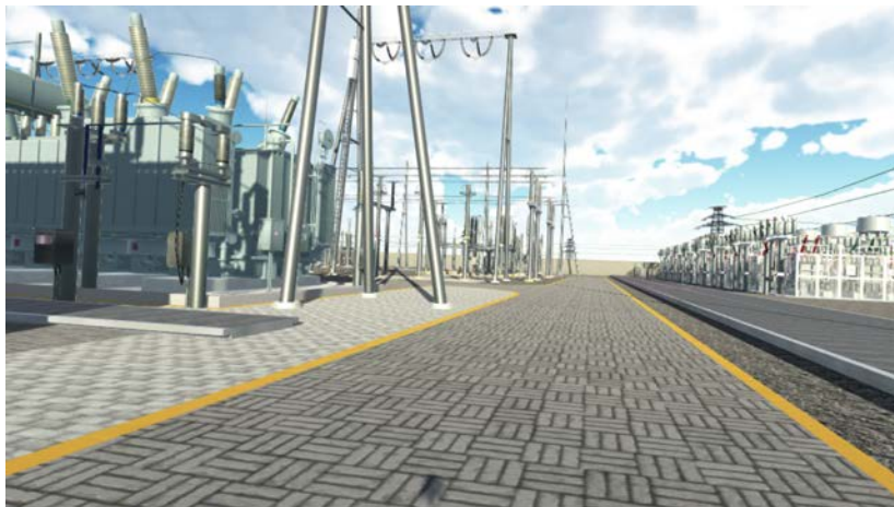
Fig. 2: The cognitive training scene of power line substation.
